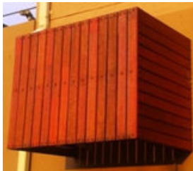
Timber and Steel Air Conditioner Covers/Screens
