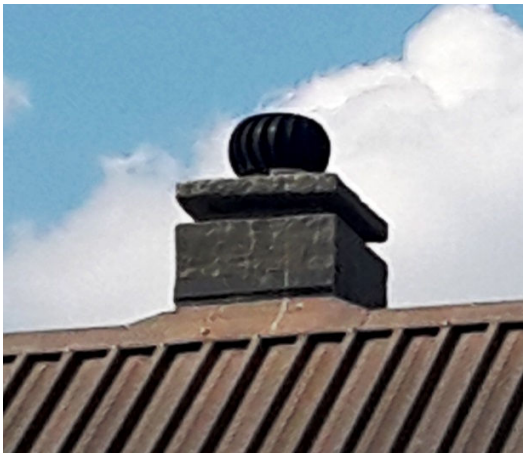
Matt Black "Tornado"/"WhirlyBird" extractor mechanisms
