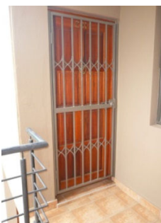
Security Doors to front doors
