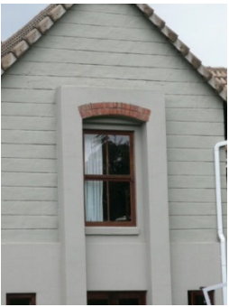
Typical External Wall finish to Second Level
