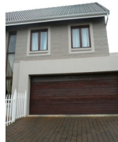
Typical Garage Door
