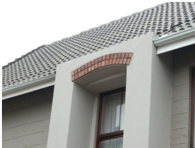
Red Face Brick Plinths
